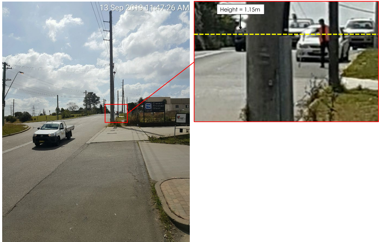
Figure 7: Sight Distance Assessment – Left-side Approach (83m at a height of 2.5m)
